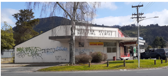
Figure 3: Vandalism on the side of the shopping centre on Brookland Road.
